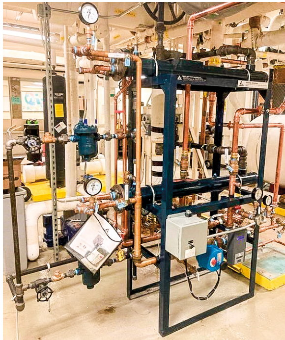
Nassau Life Insurance Company Domestic Hot Water Steam Heat Exchanger
